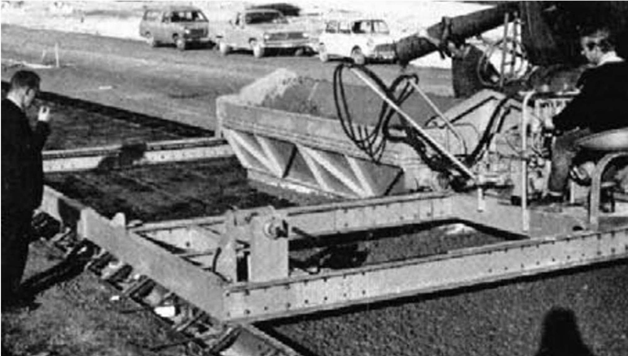
Spreading first 100mm of concrete base
