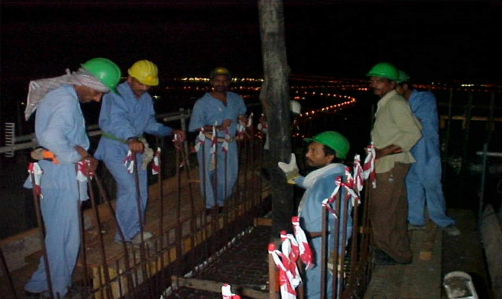
SCC pour in progress for transfer beam, Shangri-La Hotel in Dubai - 2002
