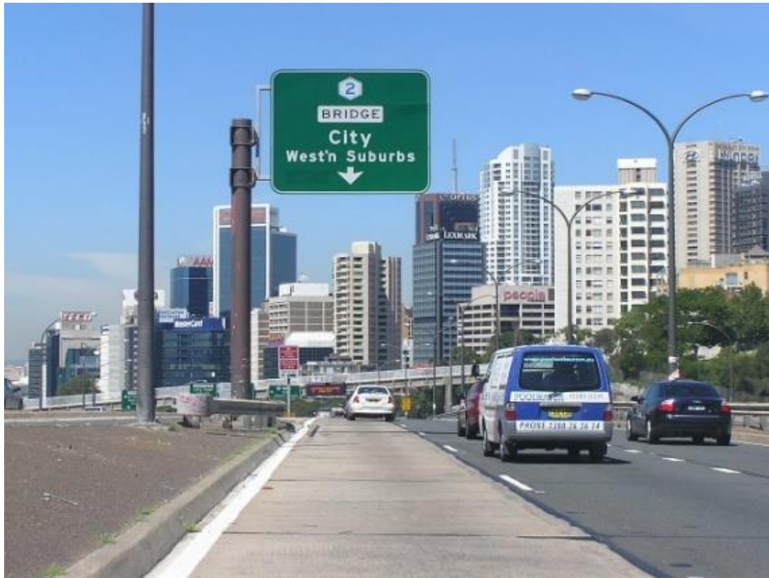
Figure 7: Concrete shoulder transformed as a travelling lane
