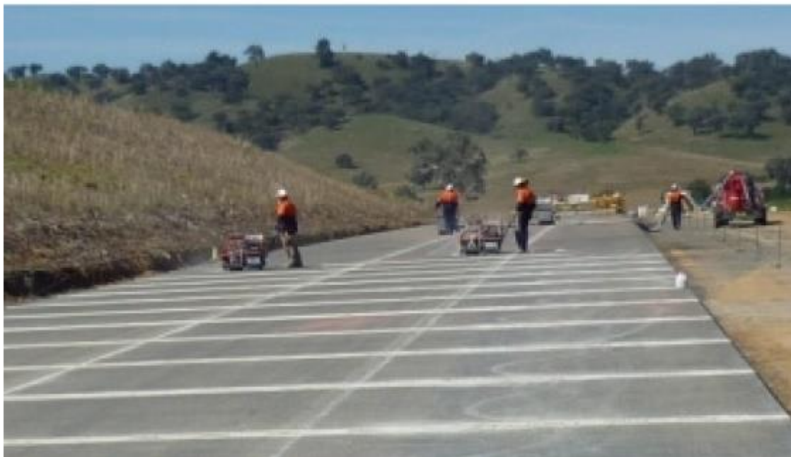
Figure 19: Transverse and longitudinal joint sawcutting in progress
