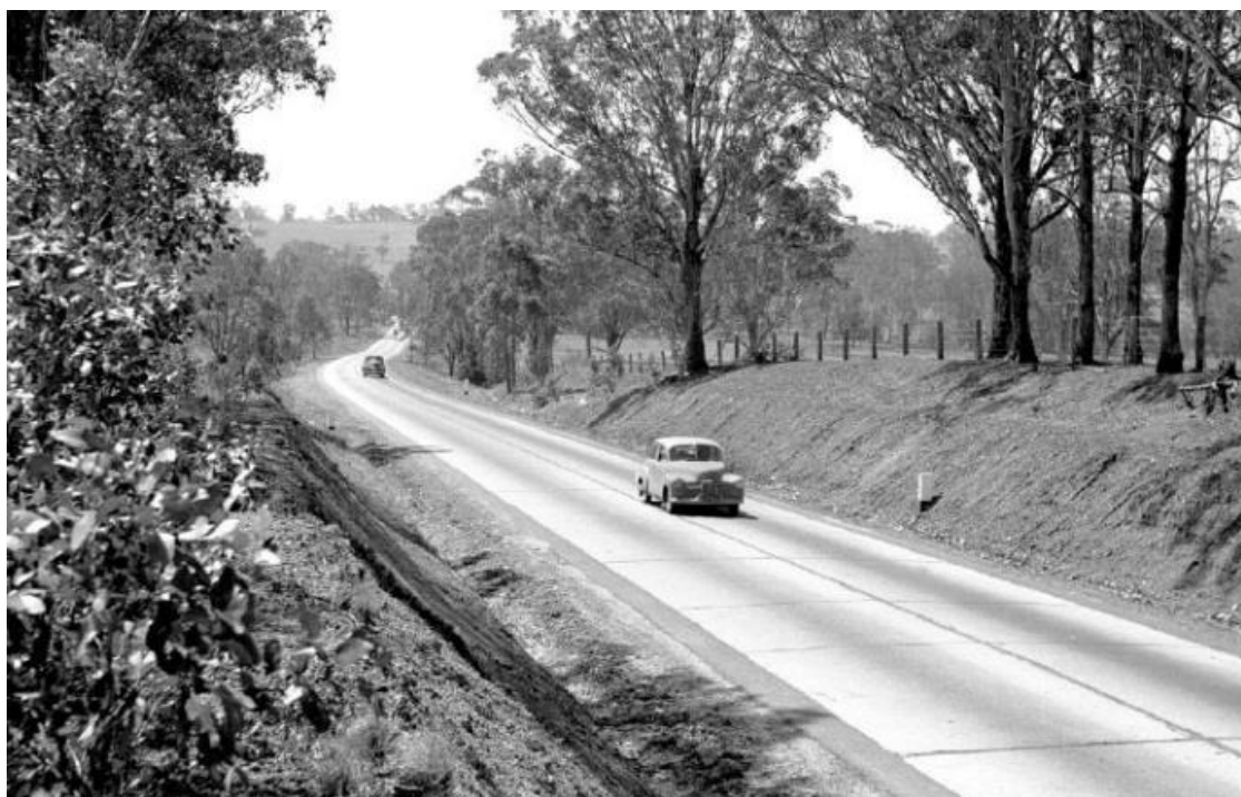
Figure 2: Sydney - Melbourne highway approximately 65km south west from Sydney (Narellan). Constructed around 1950, this highway was realigned during the 1960s/1970s
