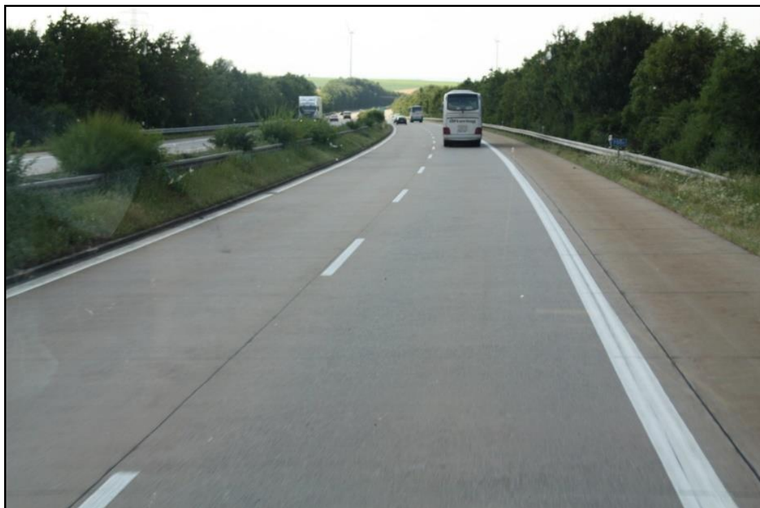
Figure 12: (b) German Autobahn A7 E45 E43 Wurzburg to Rothernburg - Constructed structural concrete shoulder and widened truck lane
