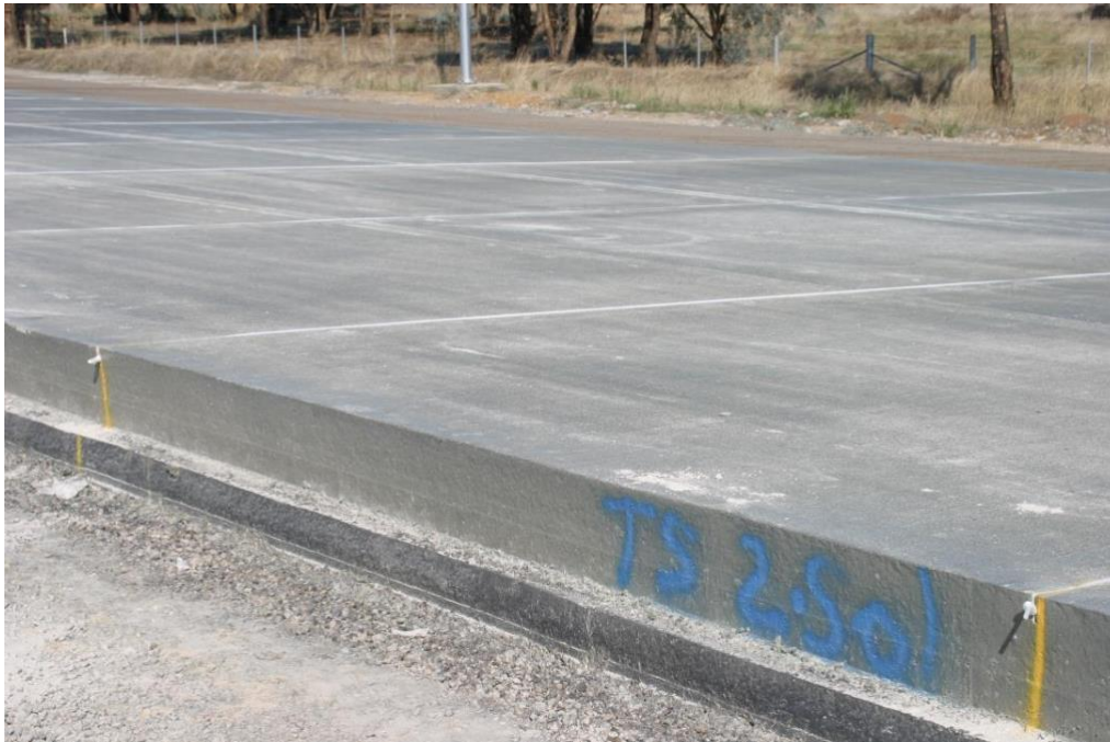
Figure 16: Completed carriageway showing additional subbase width (Fig11)
