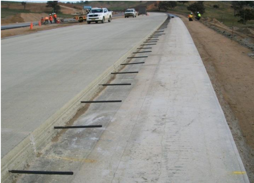
Figure 14: Completed travelling lanes with tied construction joint awaiting shoulder paving.
