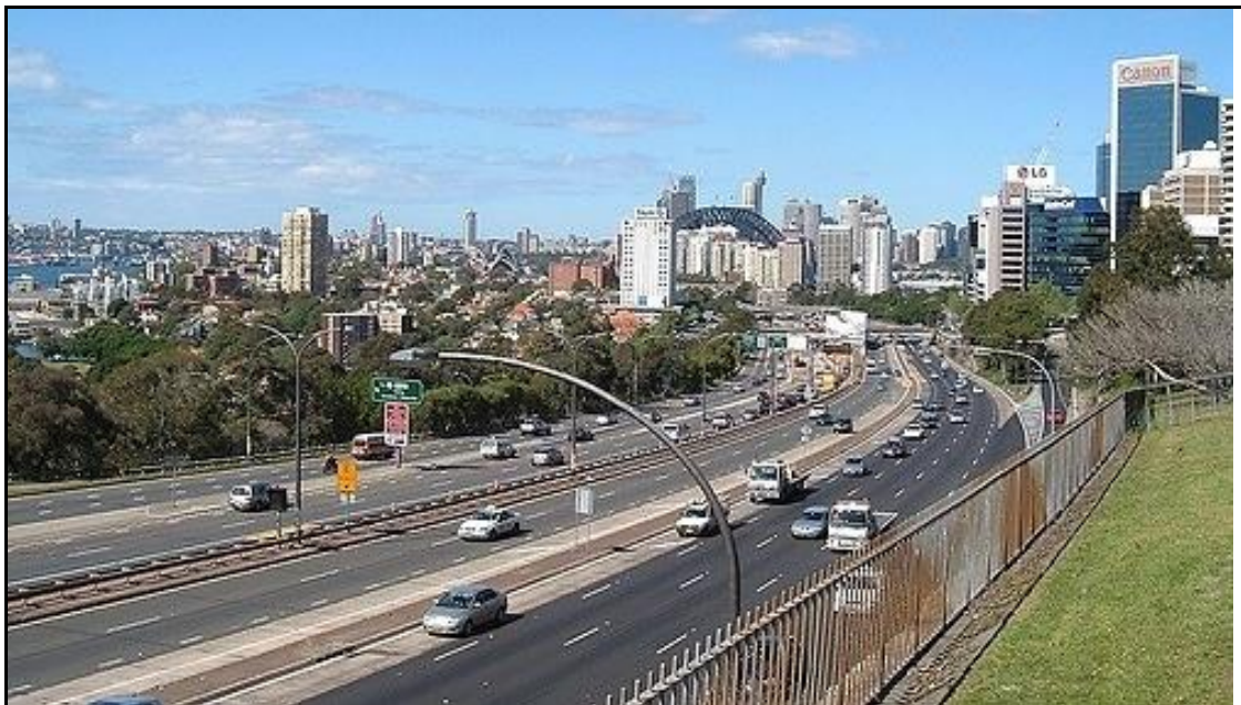
Figure 6: Concrete shoulders transformed for use as a travelling lane
