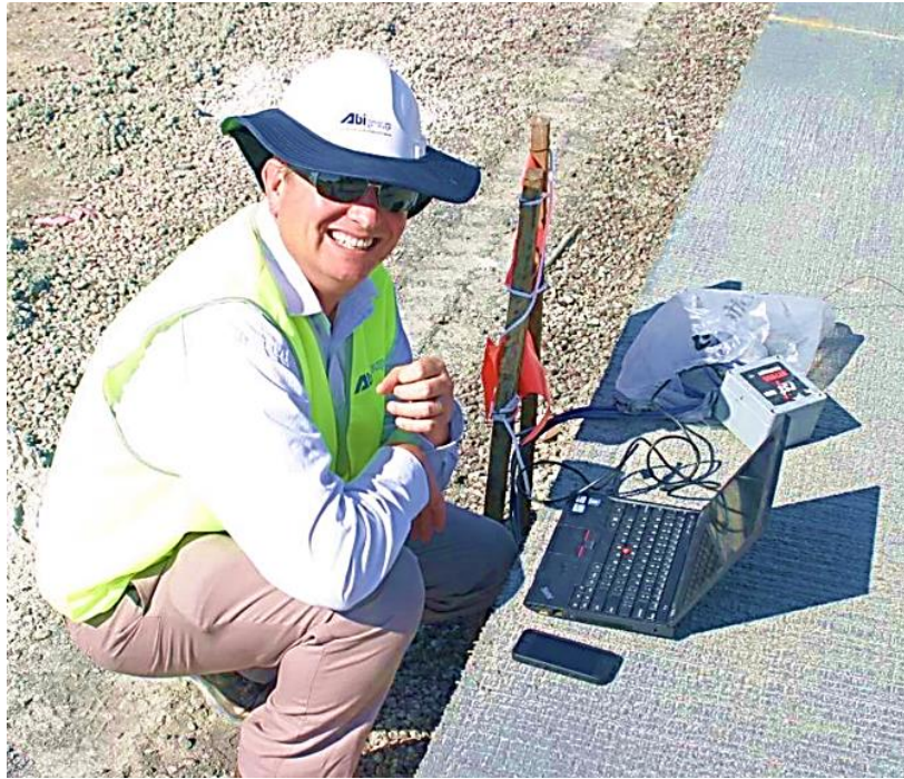
Figure 221: (b) Downloading strain gauge instrumentation data Egan (19)
