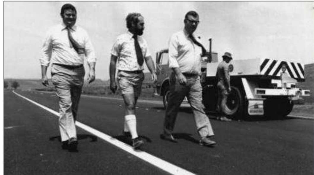
60010023 ex Blacktown, SIM SPITAL, Pix B.Gilgour. Story S.Moloney. The DMR's assistant PR officer, Bob Dudley (left) looks over the new thermo-plastic road mark markings on the new section of the F5 freeway with works engineer Lew King and regional engineer Arvo Timm.
