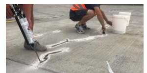
Epoxy Resin Treatment
