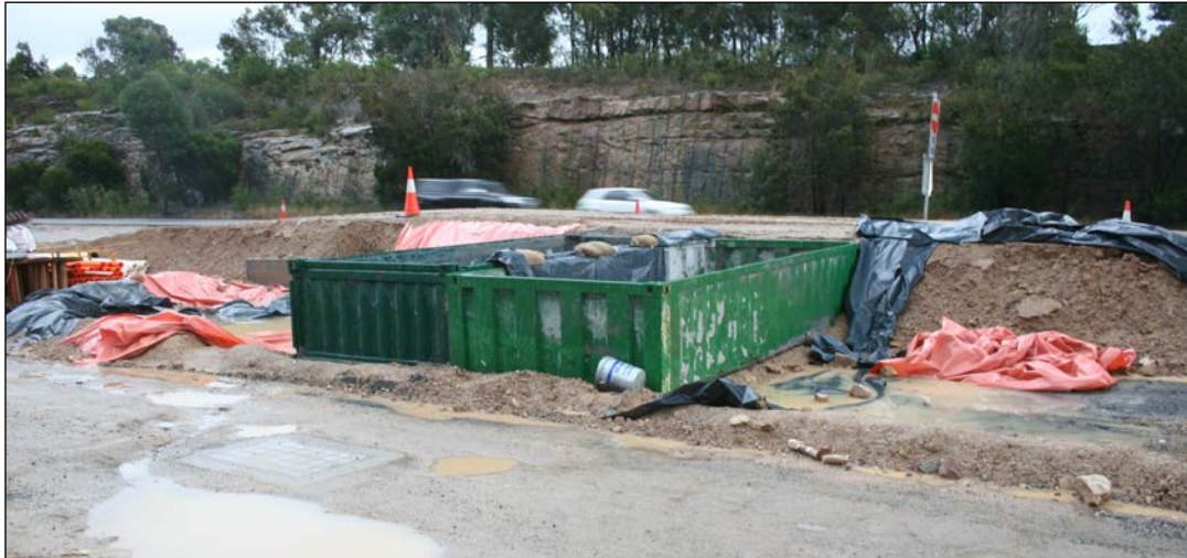
Figure 16. The construction of slurry settling ponds used on the M1 project in 2010.
