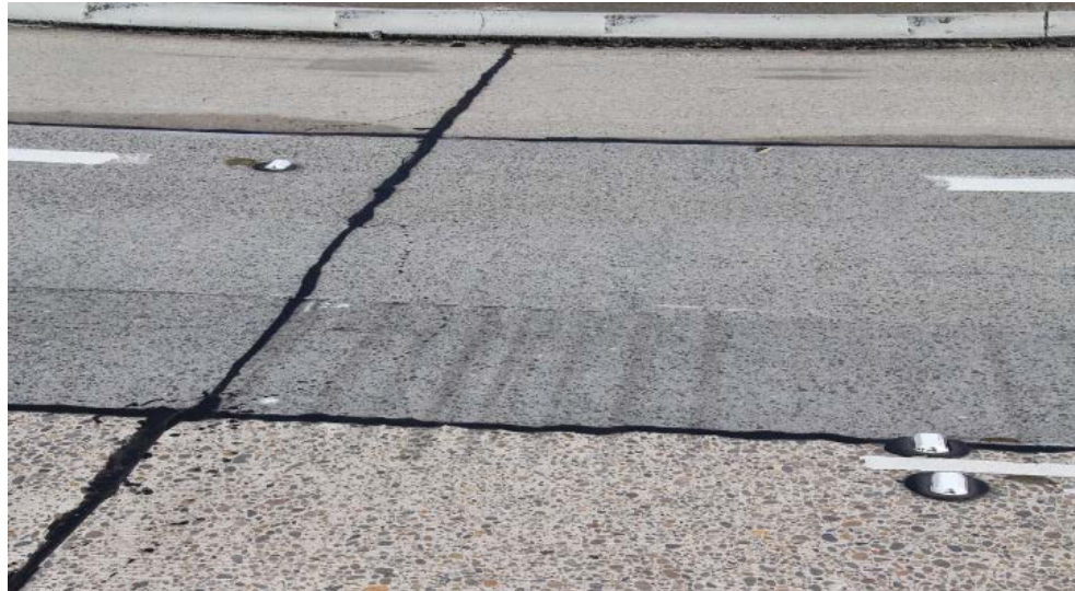
Figure 17. Nonconforming troughs in the surface caused by ‘drum hopping.’
