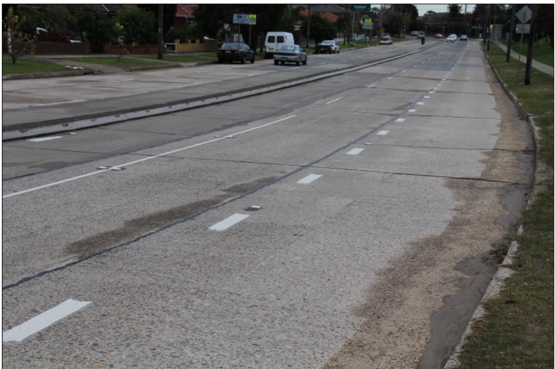
Figure 12. Conventional grinding equipment can only get to 600 mm to the edge of the kerb.
