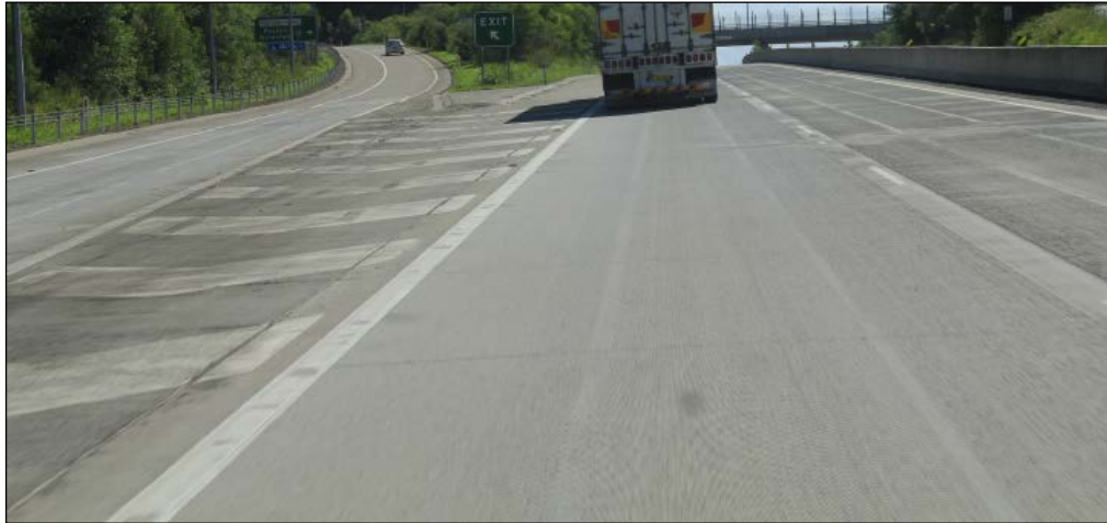
Figure 11. Overlapping run adjacent to the longitudinal joint on PCP.
