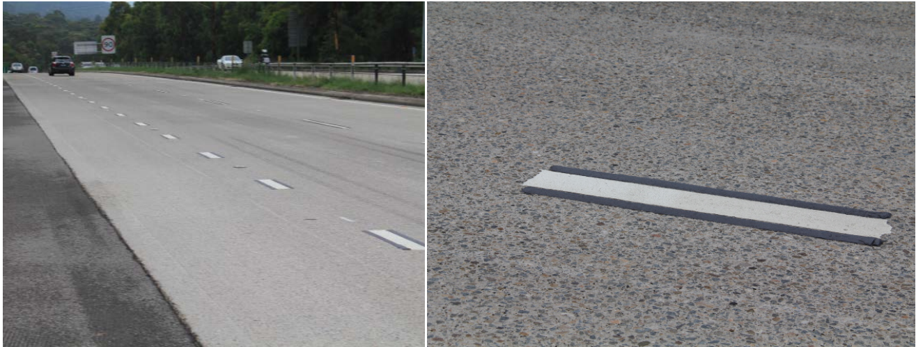
Figure 18. View of black paint applied to the concrete surface before white line marking paint is applied.
