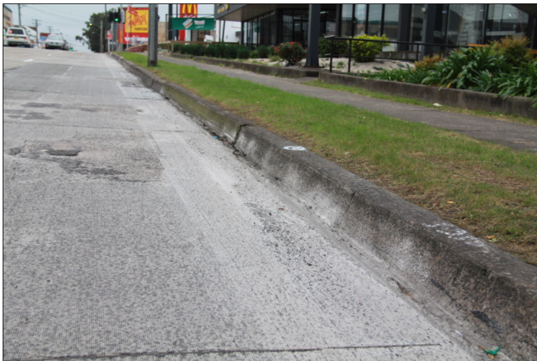
Figure 13. Grinding can be carried out close to the edge of the kerb with an attachment to the equipment.
