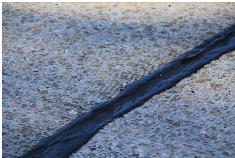
Figure 15. A bitumen emulsion seal poorly applied after grinding.
