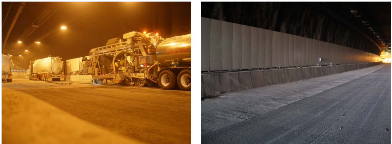
Figure 27. The diamond grinding technology has been used in the Clem7 tunnel. (Photo courtesy of Seovic Civil Engineering)
