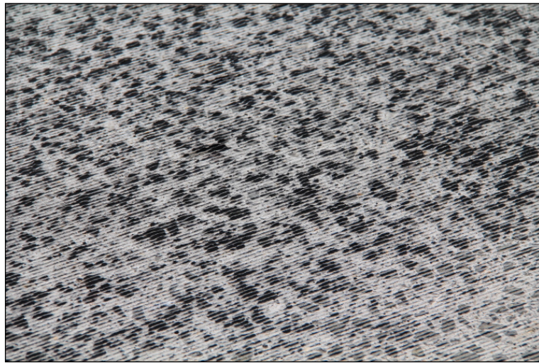
Figure 9. View of fins remaining on the surface of the M1 Motorway after 2 years of trafficking.
