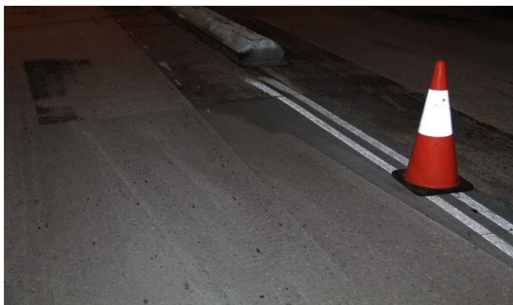
Figure 14. The grinding patch curves to match the raised median.
