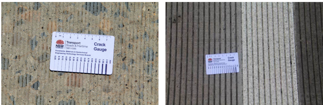
Figure 21. View of conventional (left) and low noise diamond grinding surfaces.
