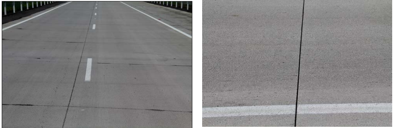
Figure 26. View of the transverse contraction joint finished with the sealant applied after grinding (left) compared with the cleaner surface appearance with sealant applied before grinding.
