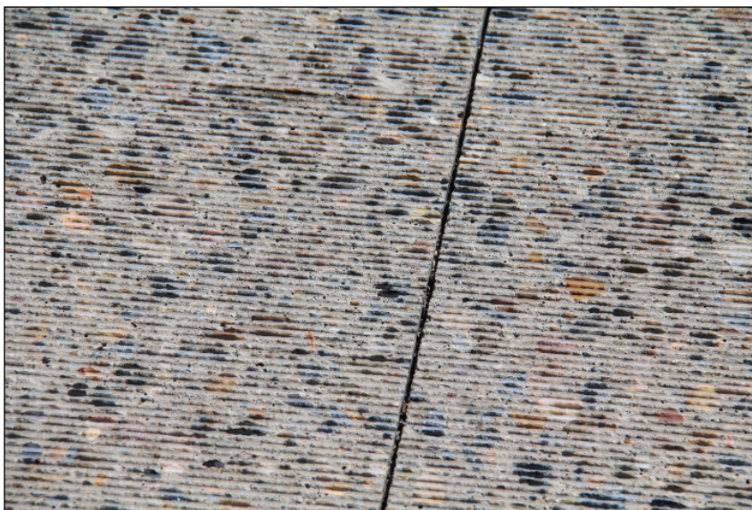
Figure 8. Surface of diamond grinding surface on California highway.
