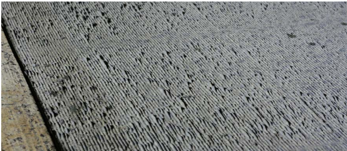
Figure 4. Grinded surface showing raised fins.
