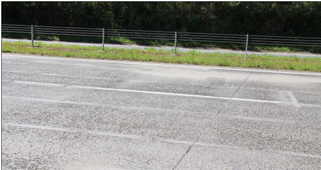
Figure 20. View of holiday (far view) commonly found at the start of slipform paving.
