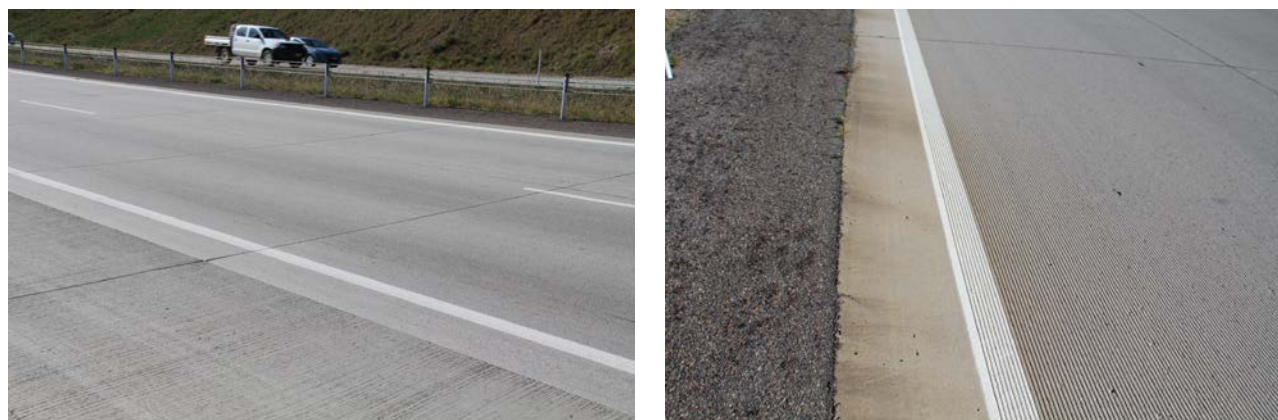
Figure 25. View of the finished LNDG surface from the longitudinal shoulder joint (left) to the outside edge of the lane marking in the median.
